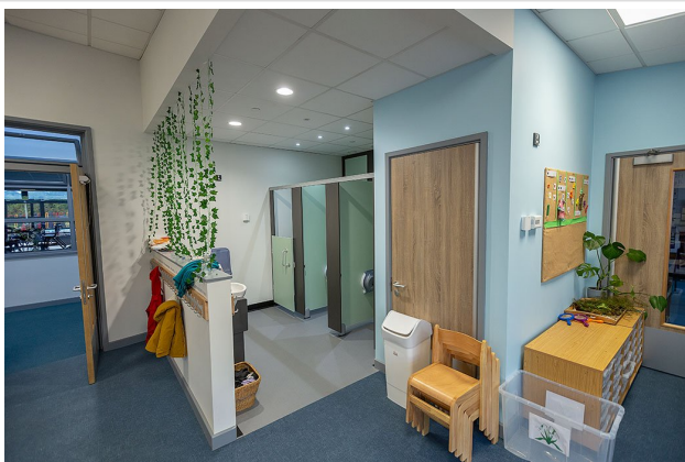
Morley Meadow using the Protec Fire Rated Downlight & BTEC
