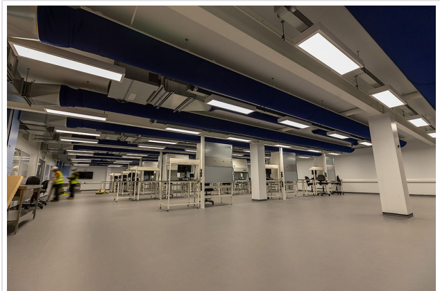
The Lighthouse Corona Testing Lab using the MODLED Suspended UGR in 1200 x 300mm
