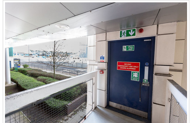
Birmingham Airport using the EXI LED
